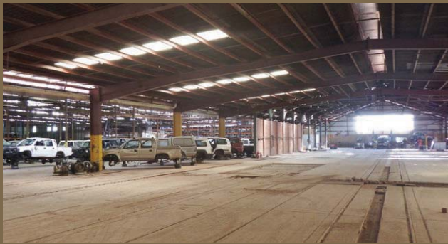
FIGURE 15: SUBSTANTIALLY COMPLIANT WORKSITE, VEHICLES PROCESSED INDOORS ON A SEALED SURFACE
