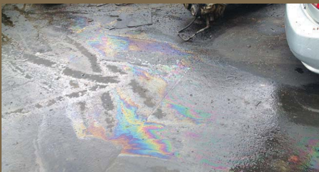
FIGURE 24: SUBSTANTIALLY NON-COMPLIANT WORKSITE, OILS AND FUELS ON GROUND CREATE A SLIP HAZARD
